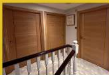
DOOR HANGING & ARCHITRAVES
