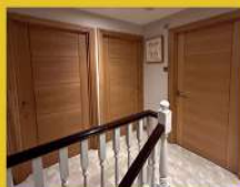
DOOR HANGING & ARCHITRAVES
